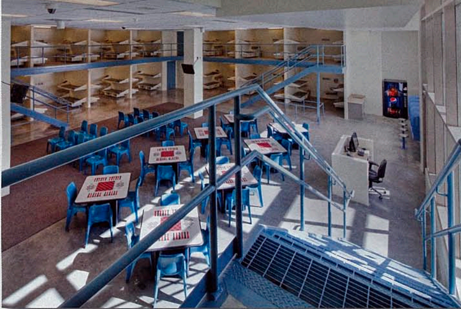
Exterior daylighting techniques may help the Van Cise Simonet Detention Center, part of the larger Denver Justice Center project, achieve LEED Silver.
